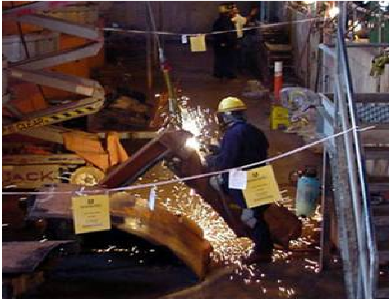
Fig. 2. Worker Using Cutting Torch
