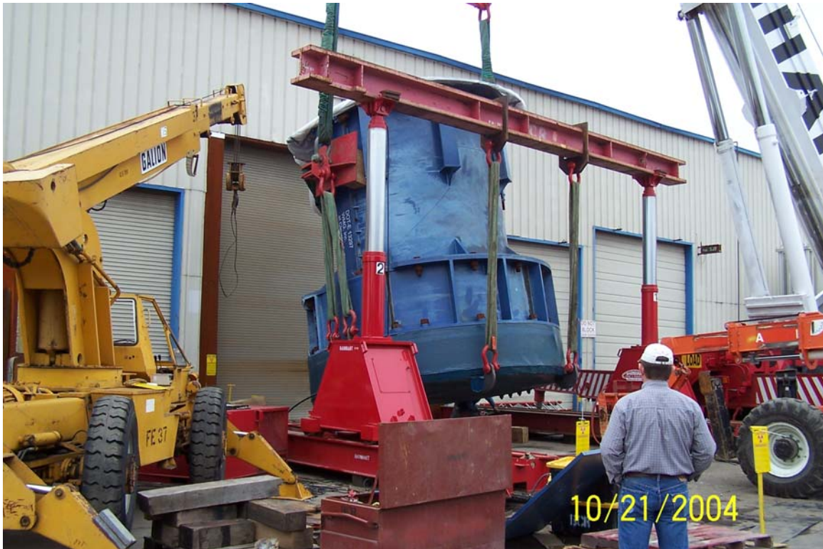
Fig. 4. Down-ending partially packaged Surry U2 head at RACE
