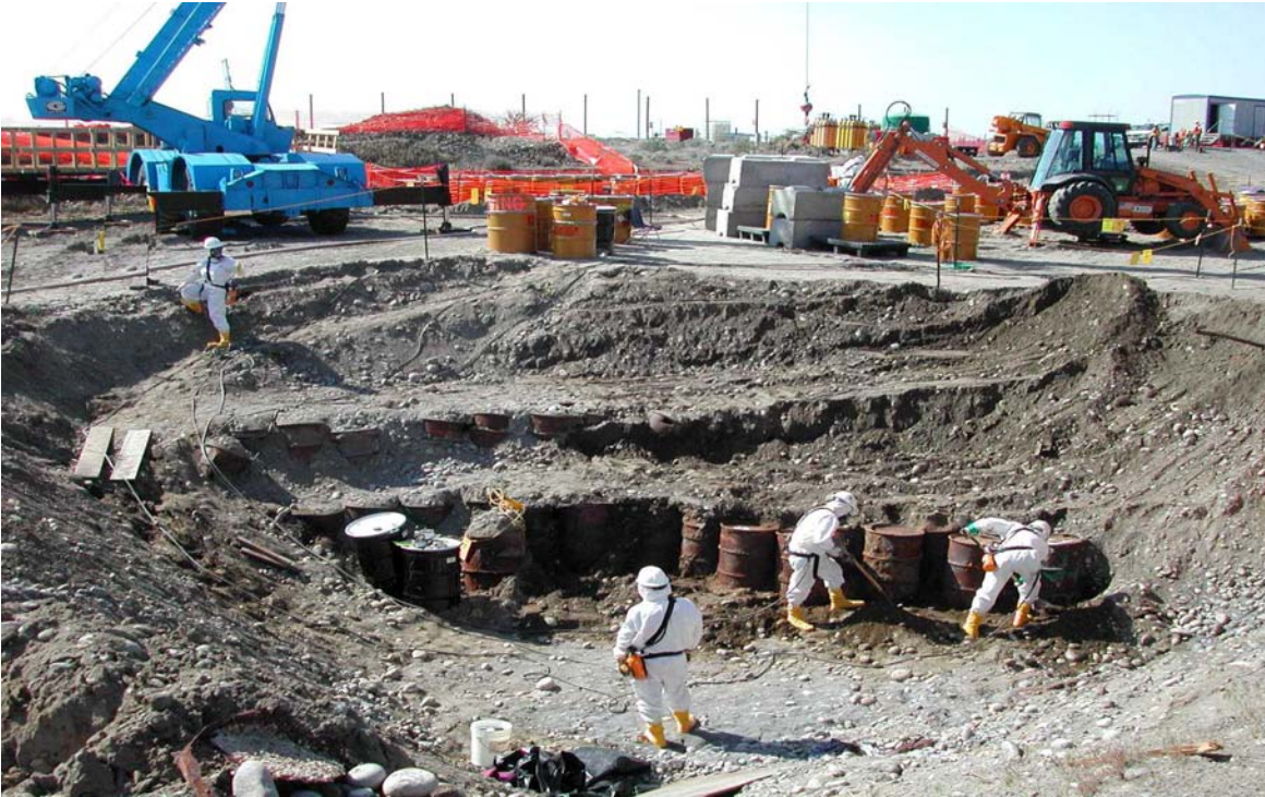
Fig. 2. Removal of Drum Containing Depleted Uranium from the 618-4 Burial Ground.
