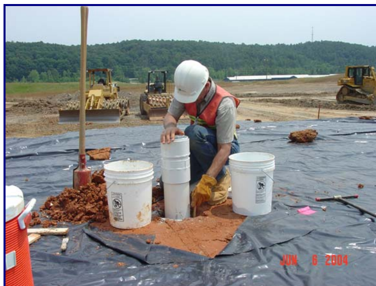
Fig. 4. Hydraulic Conductivity Testing.
