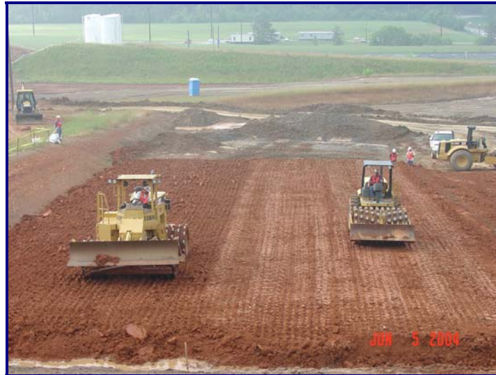
Fig. 3. Test Pad Construction and Testing.
