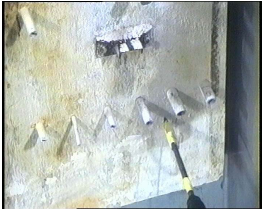
Fig. 4. Open ends of the ducts in the concrete block C 3.2
