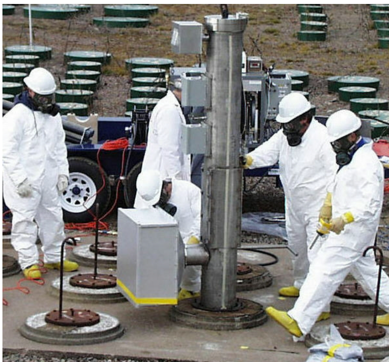
Fig. 3. Hydraulic lifting apparatus installed on tile hole.
