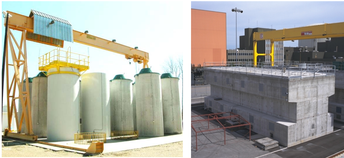
Fig. 6. Concrete Canister Storage (left) for spent CANDU fuels at CRL, and Modular Air Cooled Storage (MACSTOR ® ) module at the Gentilly-2 reactor site (right).
