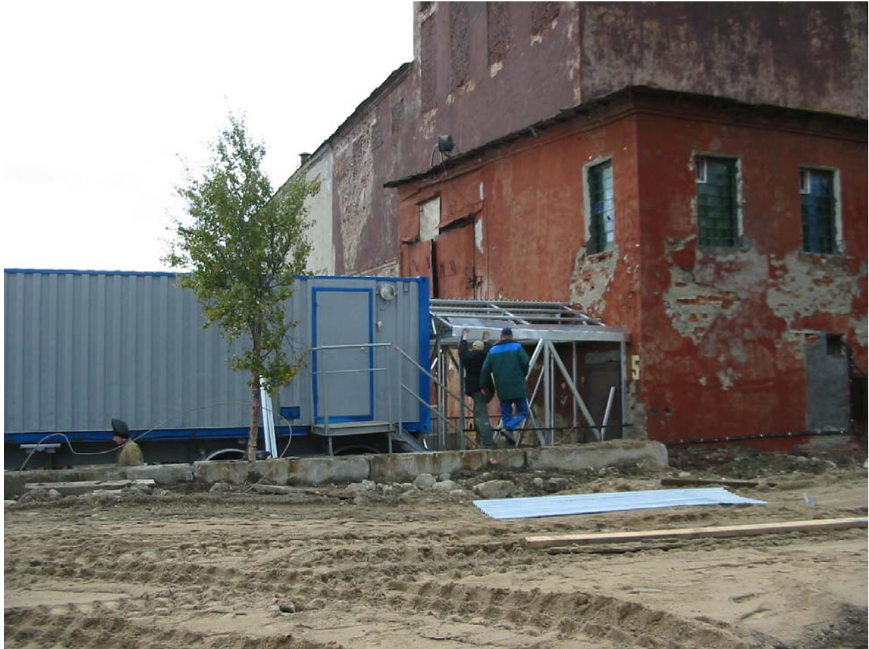
Fig. 3. Installation of the mobile sanitary pass at Building 5
