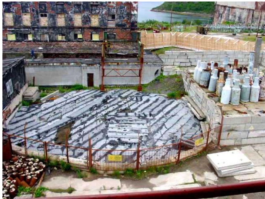
Fig. 1. Dry storage Unit 1 (facility 3A)
