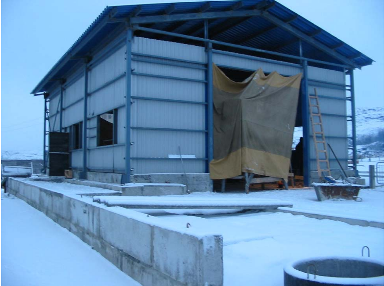
Fig. 4: The decontamination pad under construction near the SNF area.
