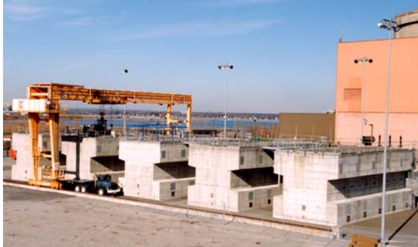
Fig. 1. MACSTOR Dry Storage Modules at Gentilly-2 in 2003. Two further modules were added in 2004.
