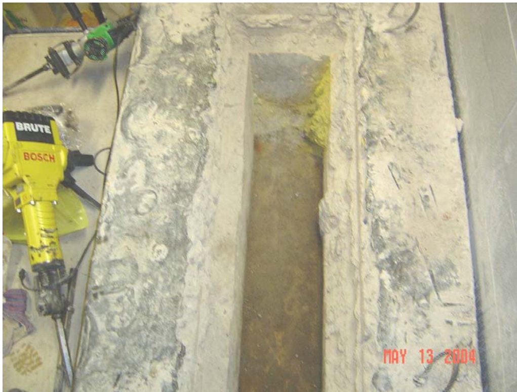
Fig. 4. All waste items excavated and removed from the vault.
