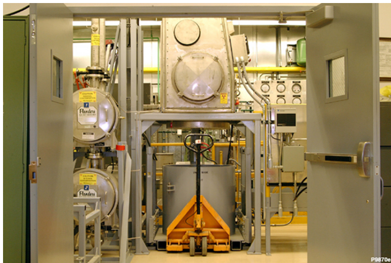
Fig. 1. SCMS solidification station.
