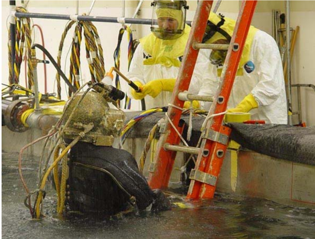
Fig. 2. Tenders spray a diver as he emerges from the water for contamination control.
