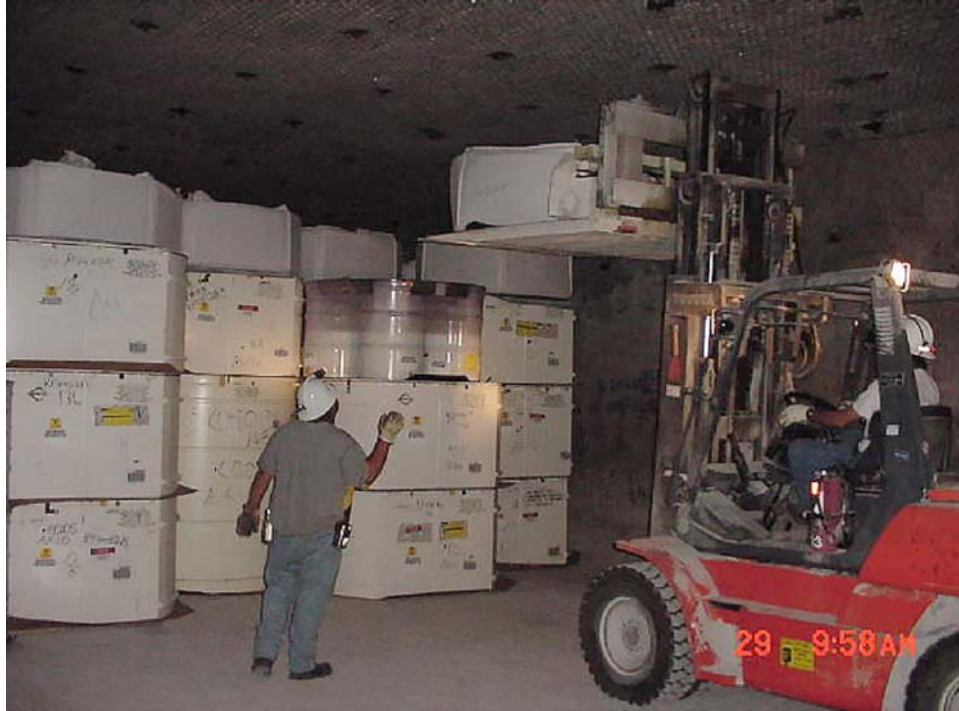
Fig. 3. MgO being emplaced on top of TRU waste at the WIPP in its underground panels.
