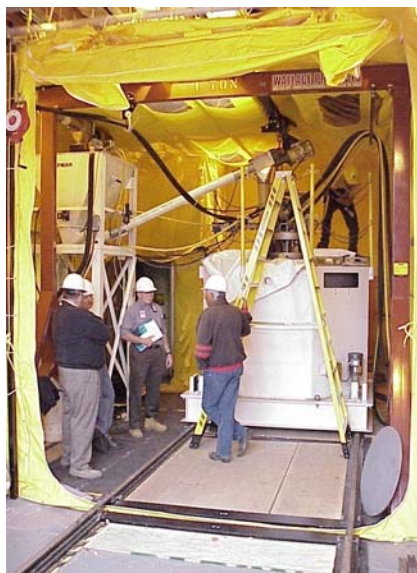
Fig. 2 . WVDP Process Area
