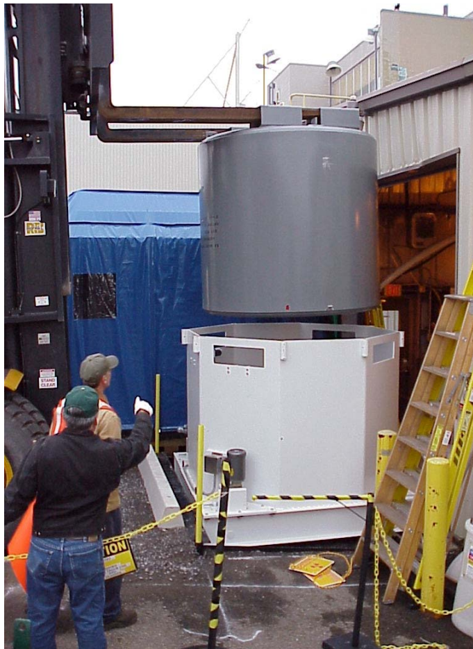
Fig. 3. Removal of Waste Container from Shield Cart
