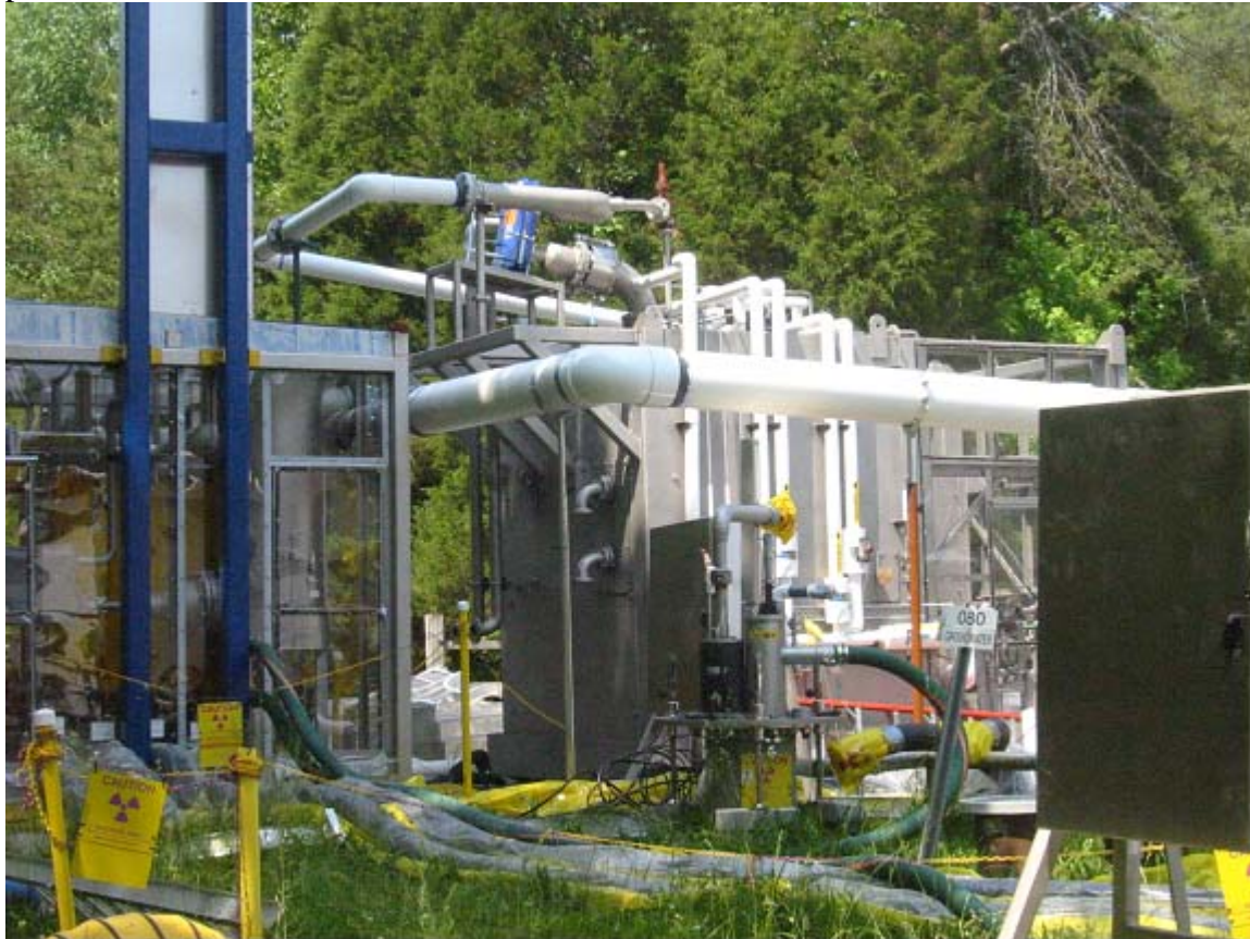
Fig. 2. The reactor module (photograph taken in Oak Ridge).
