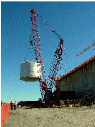
Fig. 1. Lifting a 475,000 gallon feed receipt vessel into the pretreatment facility
