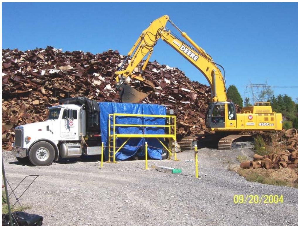
Fig. 2. Loading a dump truck
