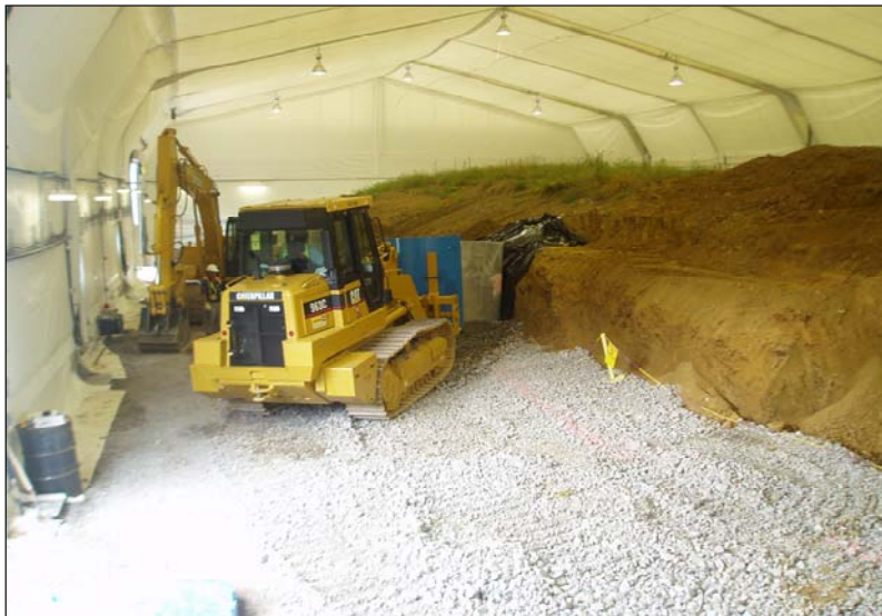
Fig. 2. Retrieval equipment inside excavation enclosure.
