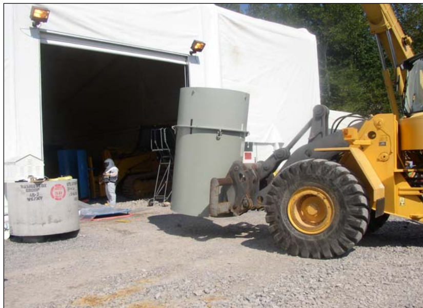
Fig. 3. Relocation of completed cask overpack.
