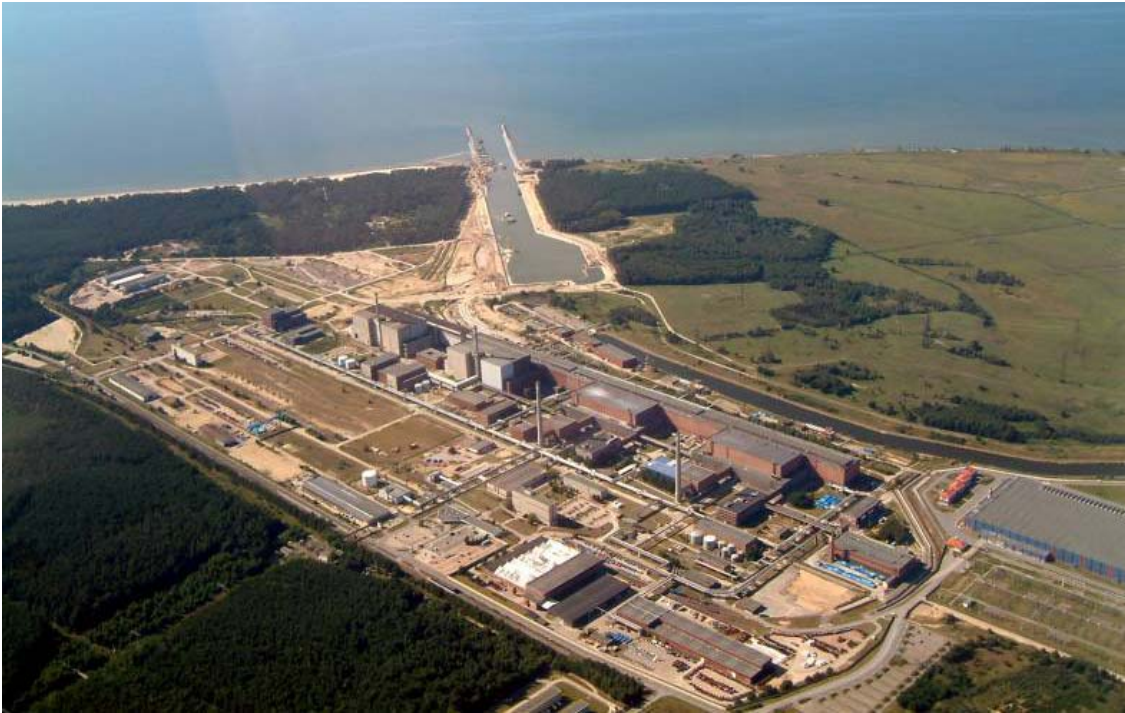
Fig. 2. Reusable properties in the left and new harbour in upper part
