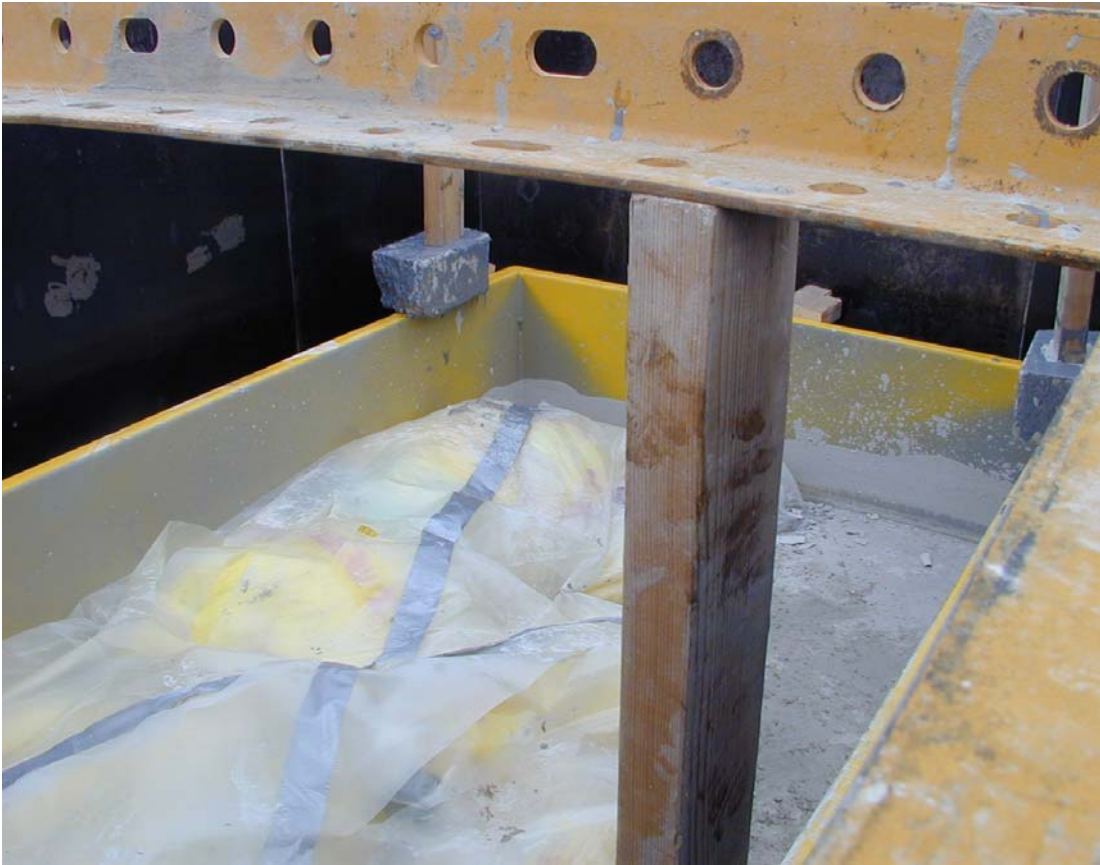
Fig. 3. Containers Staged Awaiting Macro Mix.
