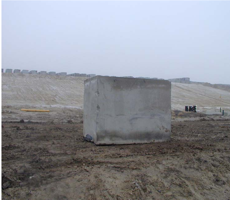
Fig. 4. Completed Macro Vault.
