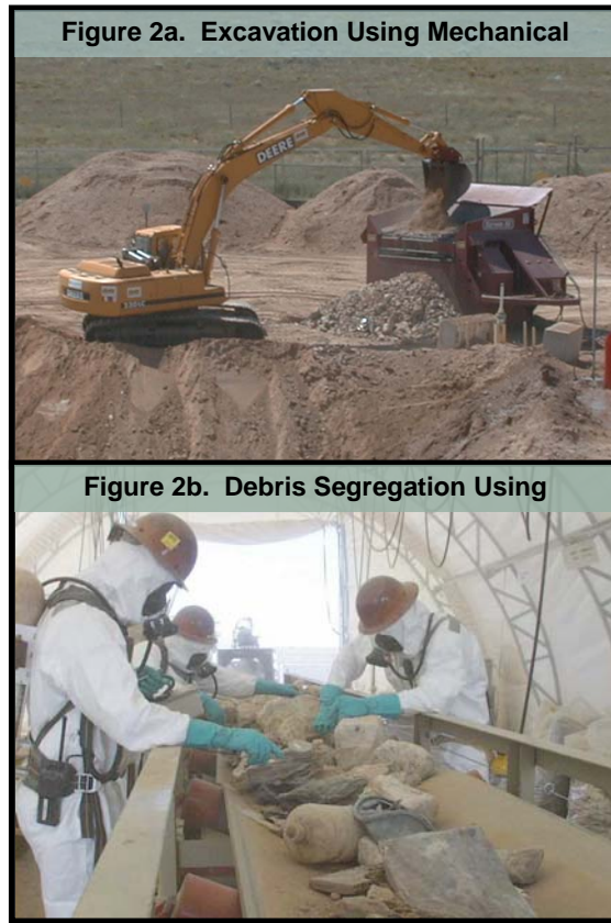
Fig. 2. Process Improvements to Excavation Operations
