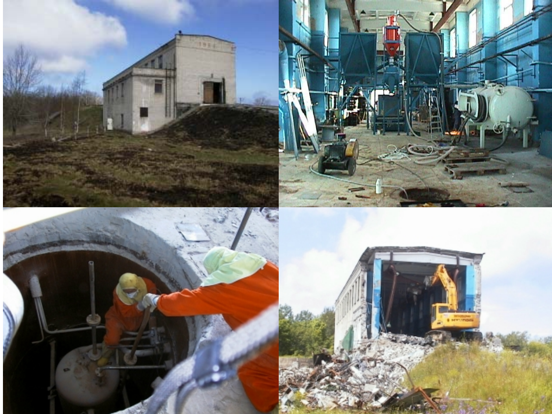
Fig. 3. The Liquid Waste Storage (LWS)
