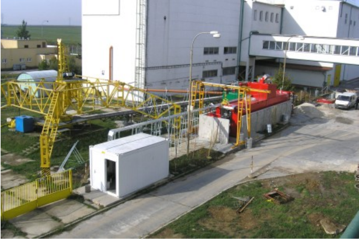
Fig. 4. Installation of the NPP at active water purification station of A1-NPP
