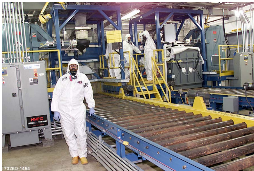
Fig. 1. Workers stand next to the Silo 3 packaging systems. On system # 1 is a Lift-liner package inside a loading frame prepared to be loaded.
