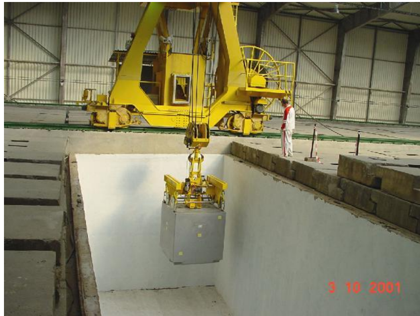
Fig. 4. Disposal of container into the concrete vault
