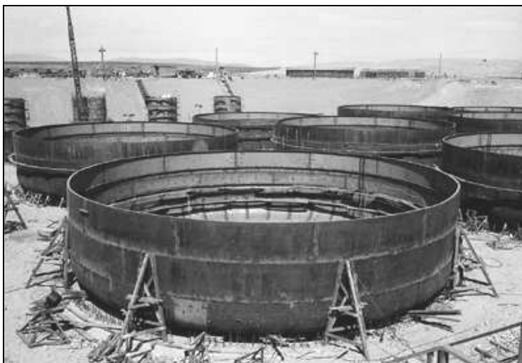
Fig. 1. One of Hanford's single-shell tanks during construction.
