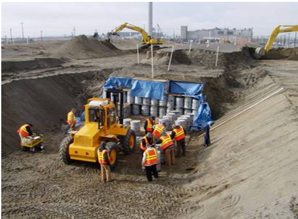
Fig. 2. Trench Excavation and Drum Exhumation Operations at 218-W-4C, Trench 4.
