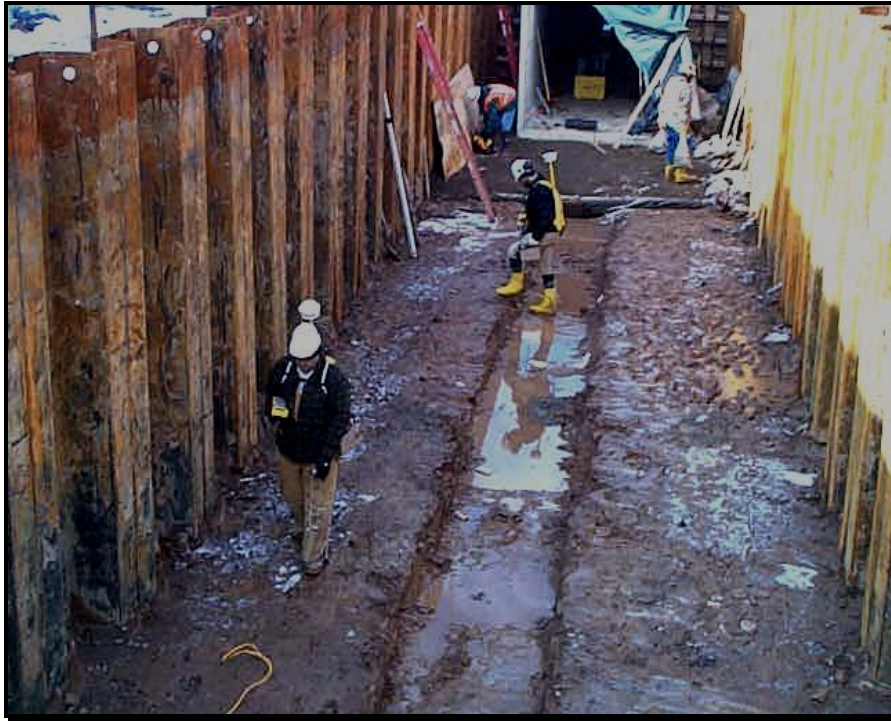
Fig. 3. Gamma Walkover Surveys Using Global Positioning Systems.
