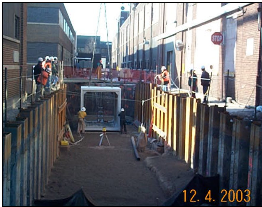
Fig. 4. Pre-Cast Box Culvert Placement.
