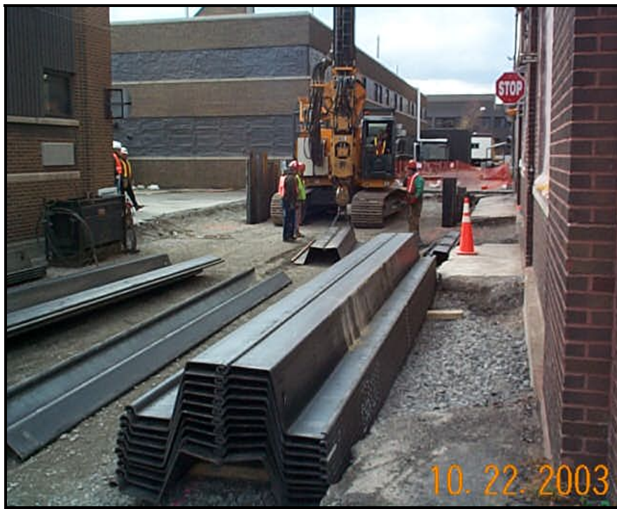
Fig. 2. Sheet Pile Installation Using the ABI Delmag TM-16 in Close Confines.
