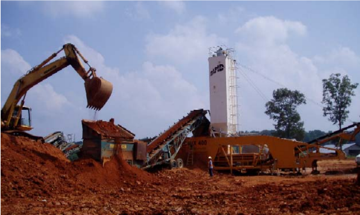
Fig. 4. Bentonite Pugmill at EMWFM Borrow Source.
