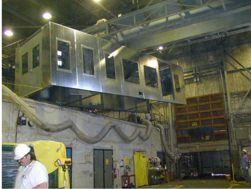
Fig. 3. Installation of the Primary Containment
