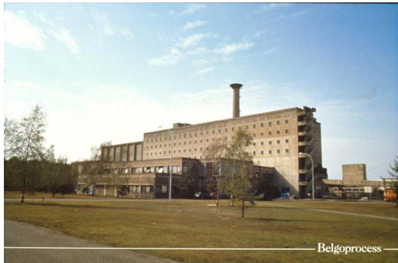
Fig. 1. Main process building of the former Eurochemic reprocessing plant
