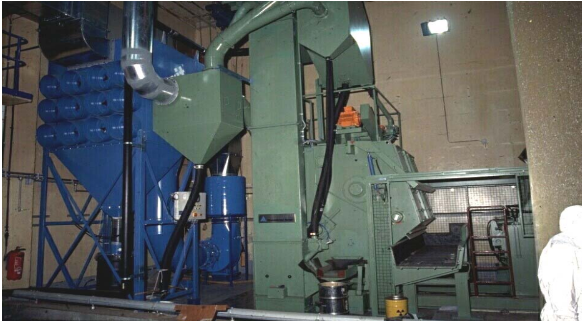
Fig. 2. Operational view of the abrasive blasting installation
