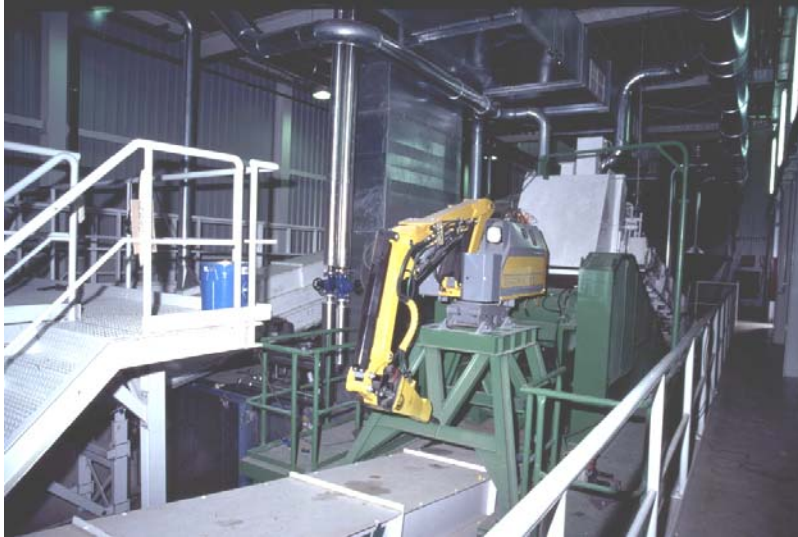
Fig. 3. General view of the concrete crushing and sampling facility
