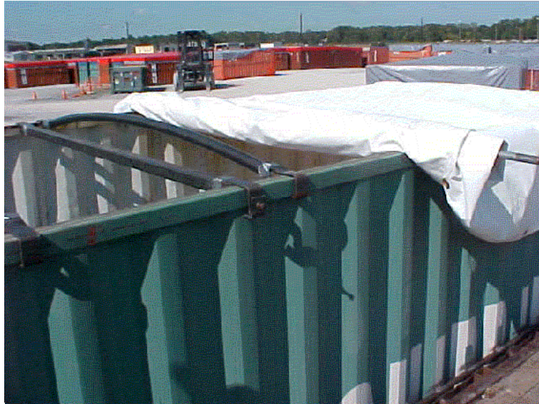
Fig. 2. Open-top view of the container from the above-grade working platform.
