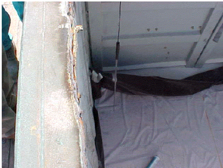
Fig. 4. Monitoring at the working level surface.
