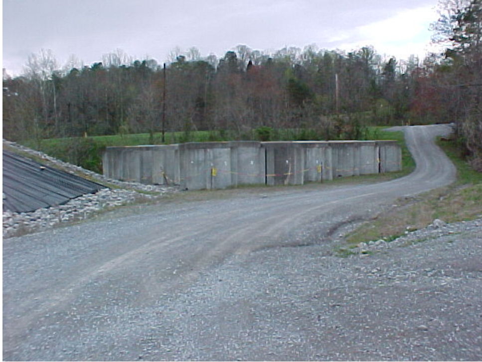
Fig. 2. Monolith casks with lids before relocation to the IWMF pad in SWSA 6.
