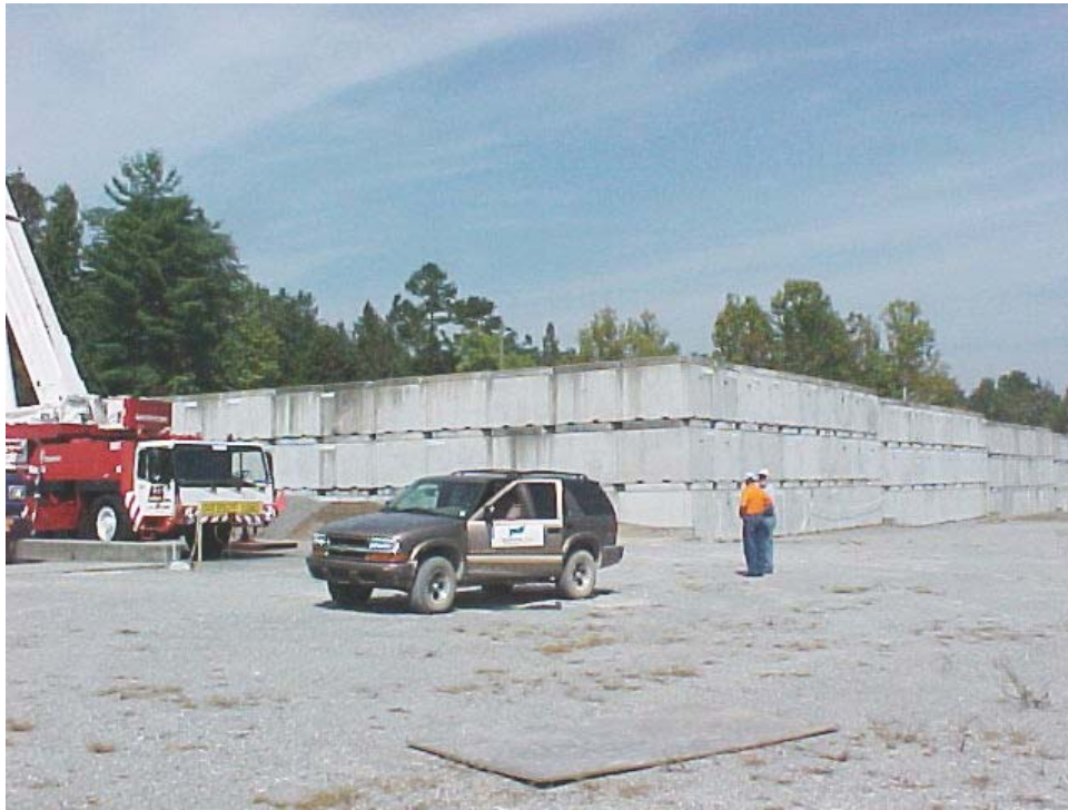
Fig. 1. Overview of the IWMF illustrating full pads containing regular vaults and a nearby empty pad with a crane readied for adding more casks and vaults.
