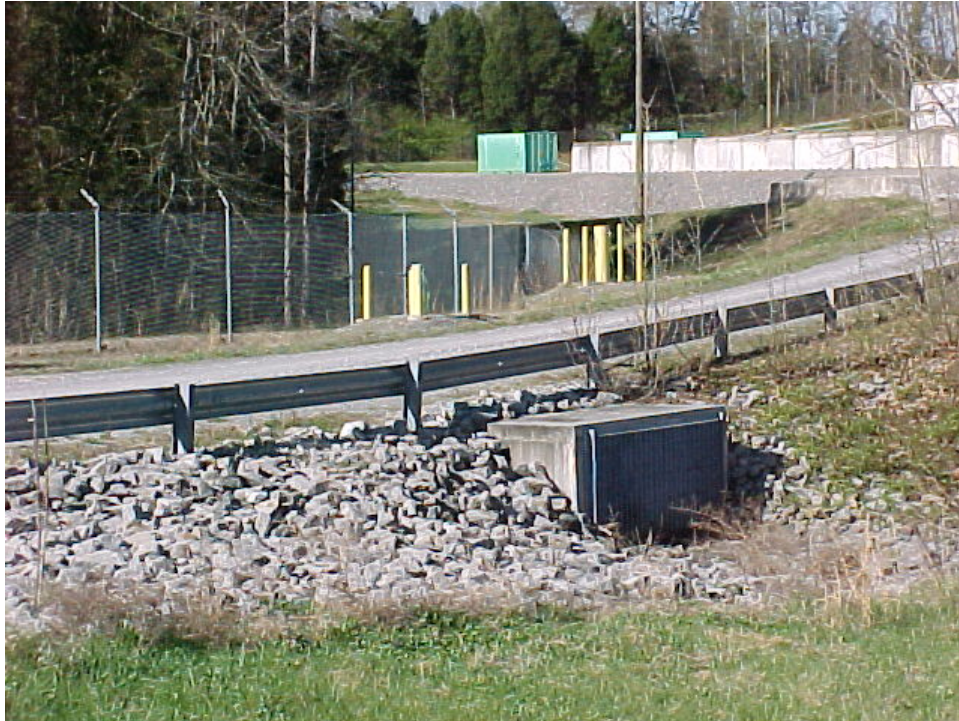
Fig. 5. Rectangular concrete culvert under IWMF Drive.
