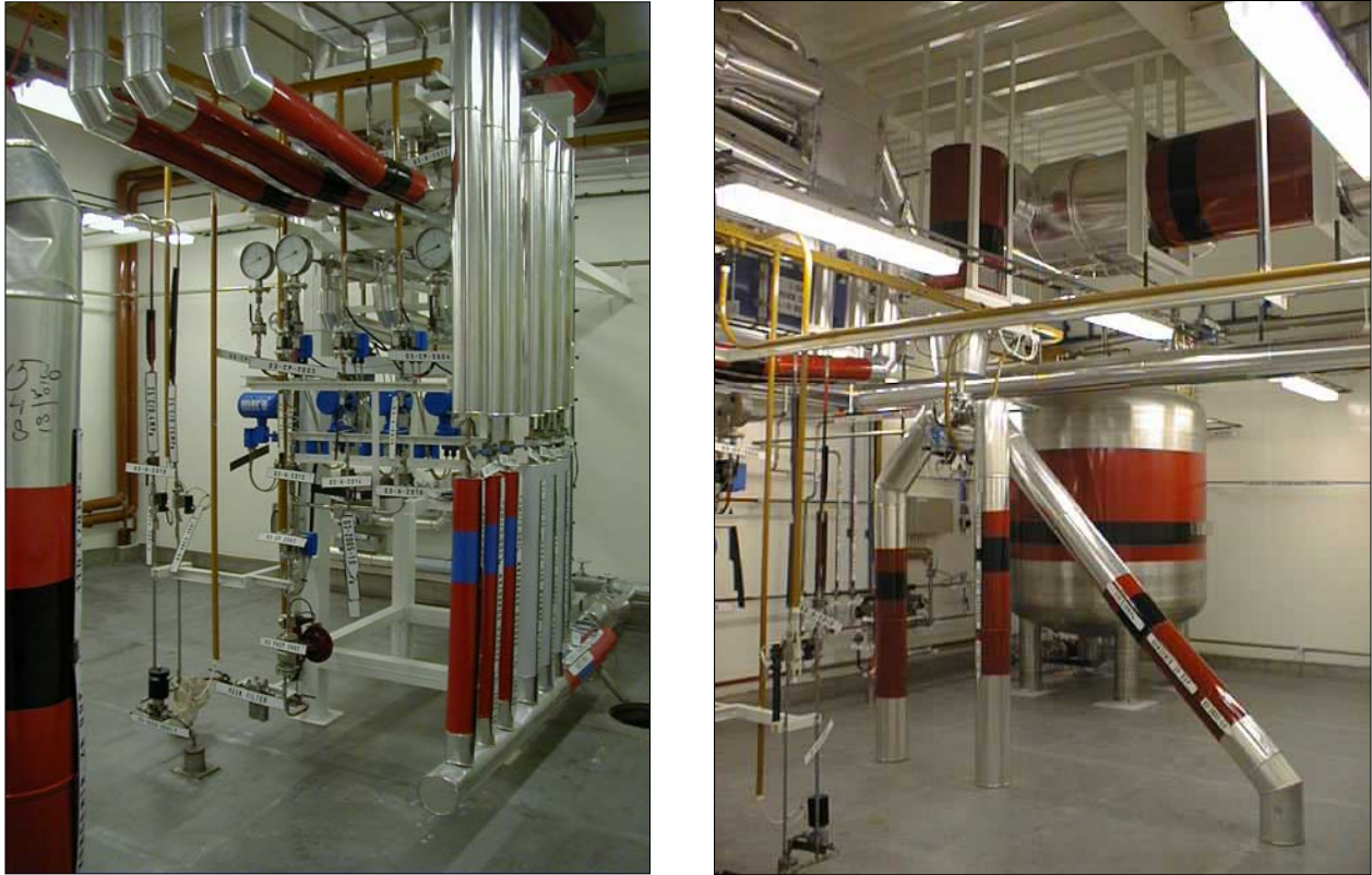
Fig. 2. UGU multi-tube hairpin heat exchanger (left) and cyclone separator (front right)
