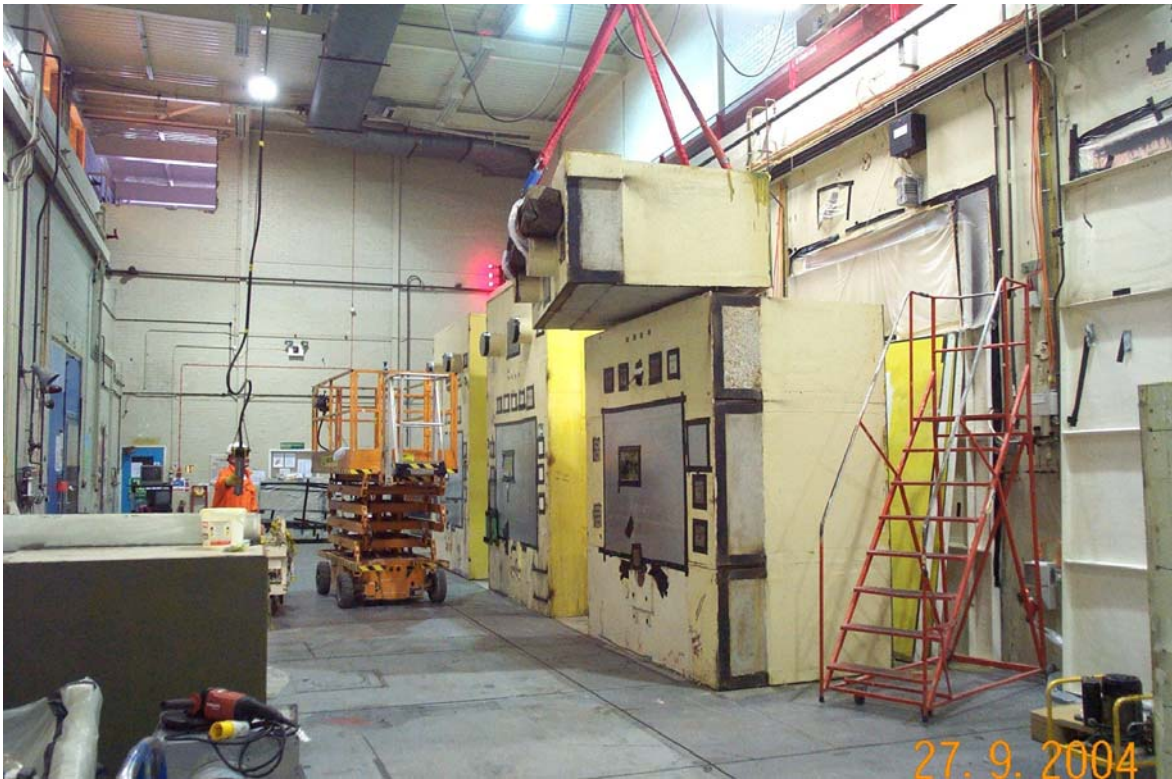
Fig. 1. Withdrawal and dismantling of the NCL window plug units
