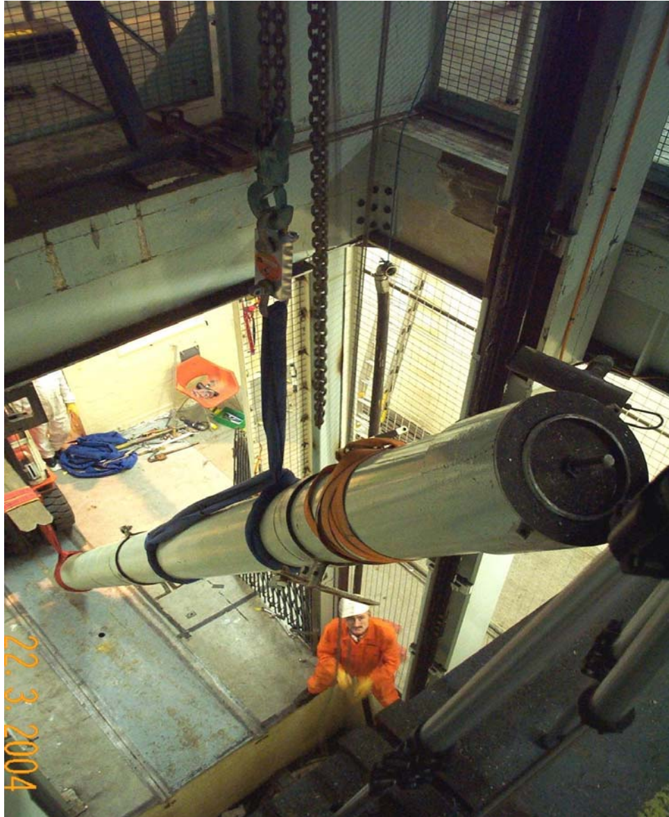
Fig. 3. Dismantling of the Pickering hoist
