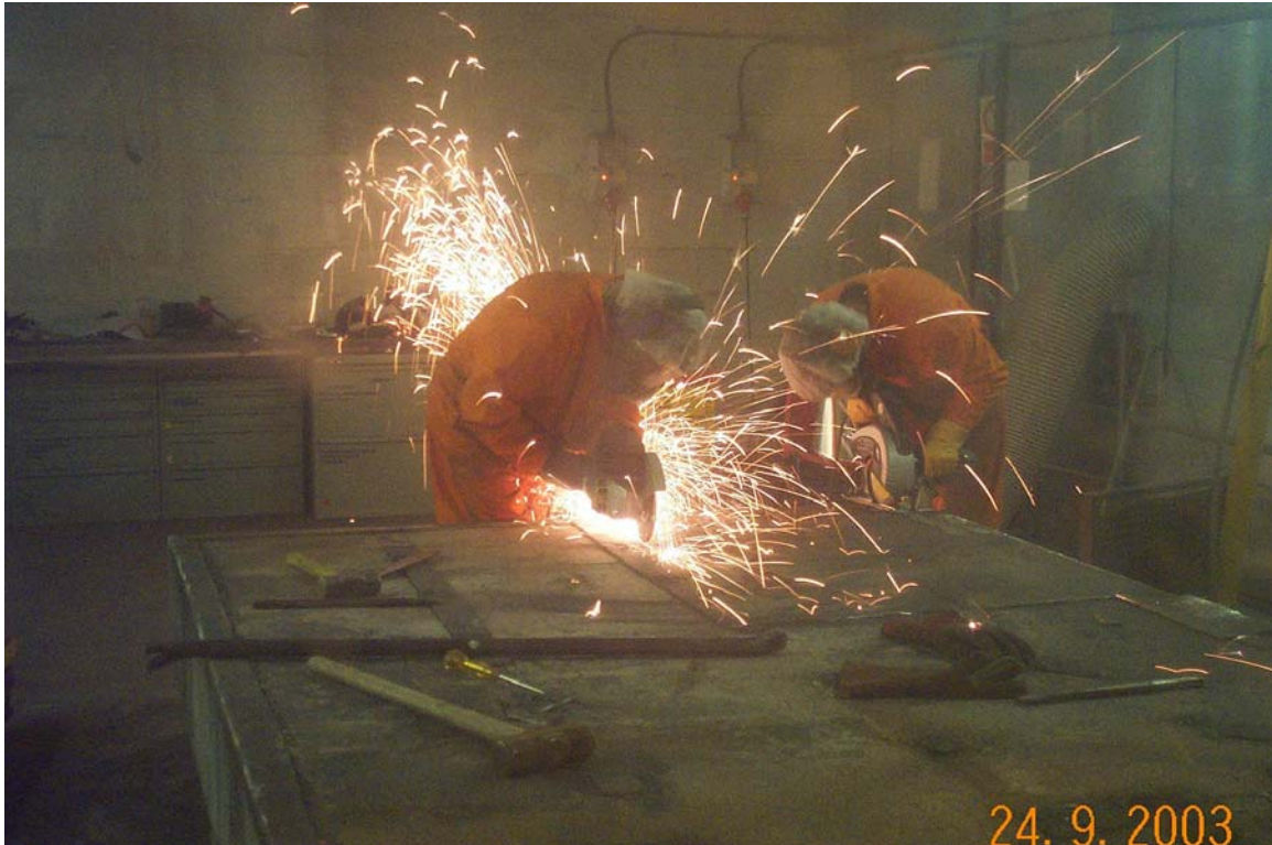
Fig. 4. Removal of steel plates from concrete blocks in the ‘Squash Court’
