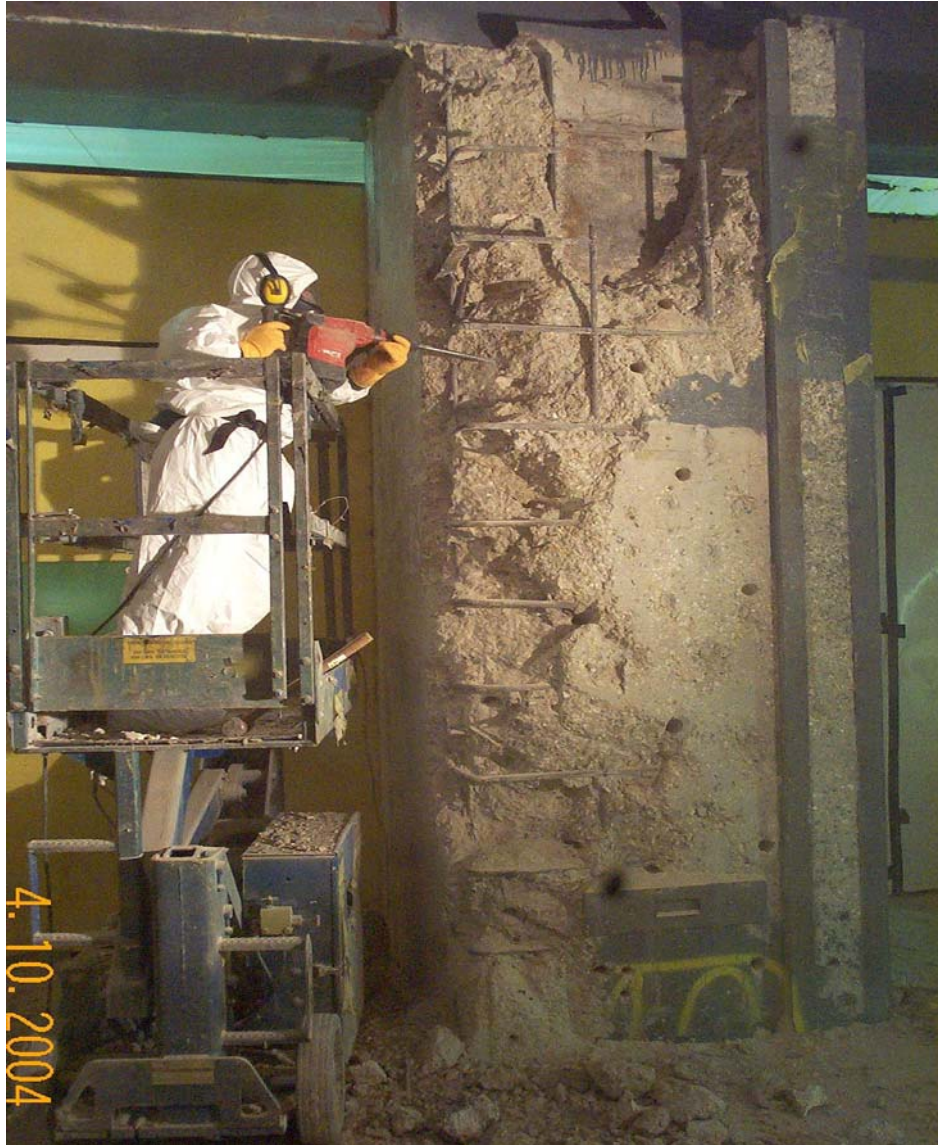
Fig. 2. Breaking away concrete from the encast ventilation ducts
