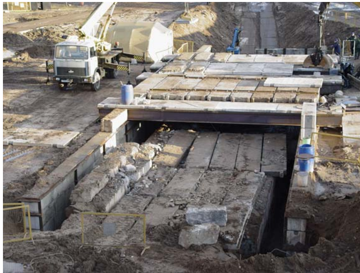
Fig. 2. Top view of the shadow shielding arrangement at repository No. 4
