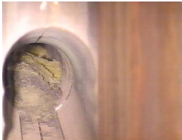
Fig. 3. Fuel element debris within FAZ fuel channel
