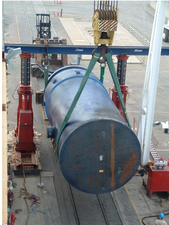
Fig. 3. Positioning Lower B SG onto QTTX Railcar.
