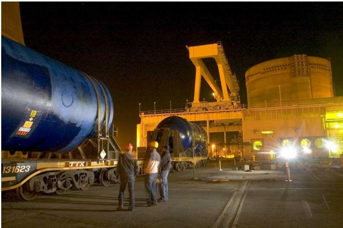
Fig. 4. SG Sections Leaving Rancho Seco.
