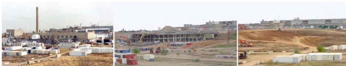
Fig. 3. Building 771 was demolished on Oct. 12, 2004. Since then, the site of the building has been backfilled, contoured and re-seeded with native grasses.
