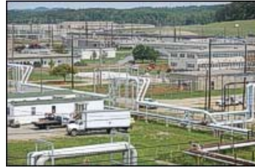
Enrichment ends; plant placed in shutdown
