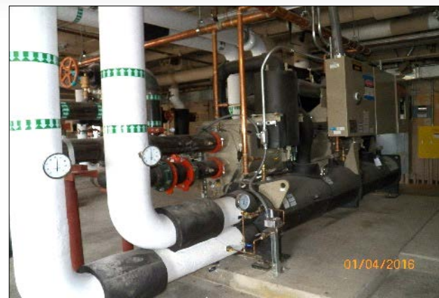
LLNL B131 Chiller Replacement
