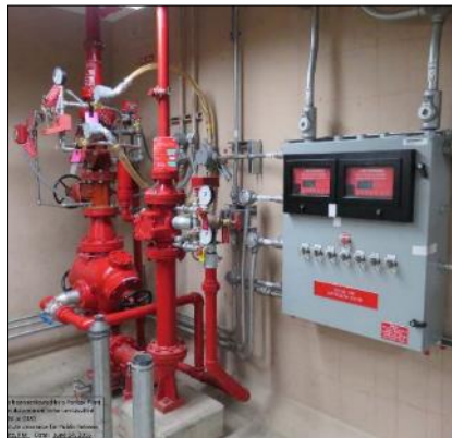
Pantex Bay/Cell and Lead In/Flame Detection System
