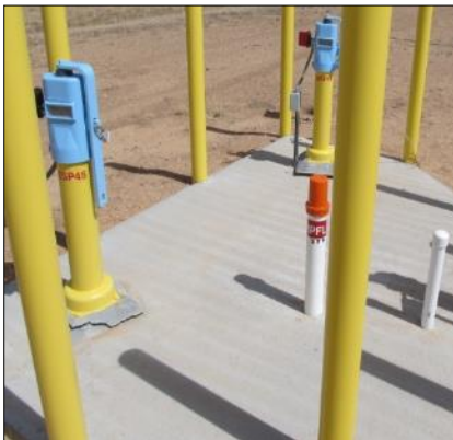
Pantex Bay/Cell and Lead In/Flame Detection System
