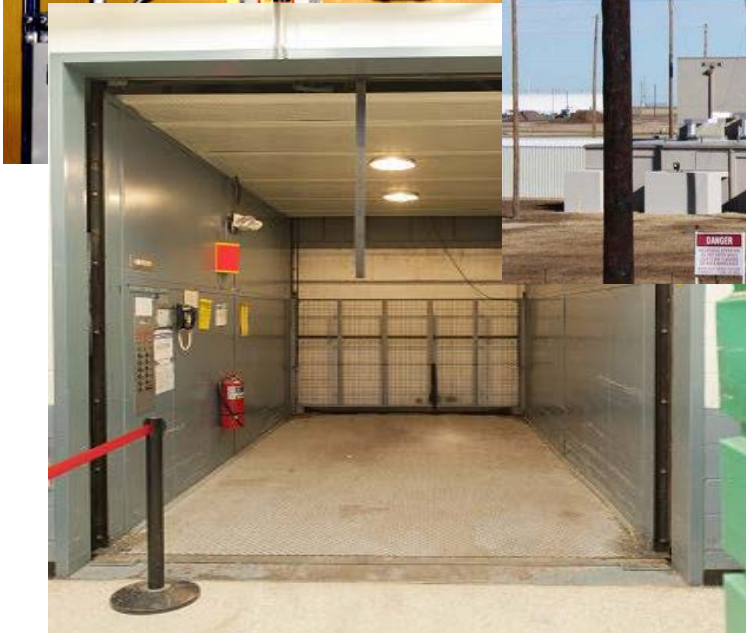
Freight elevator repairs/upgrades
