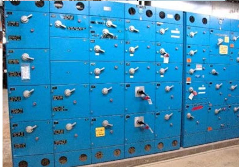
Replace distribution interconnects and motor control centers
