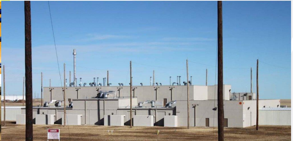
New HEPF facility
