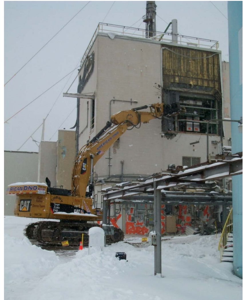
01-14 Building "Outside-to-Inside" Demolition
