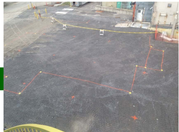
01-14 Building at Start and Completion of Demolition
