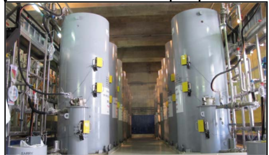
Simplified Active water Retrieve and Recovery System
