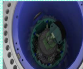
Upper CSB cutting
