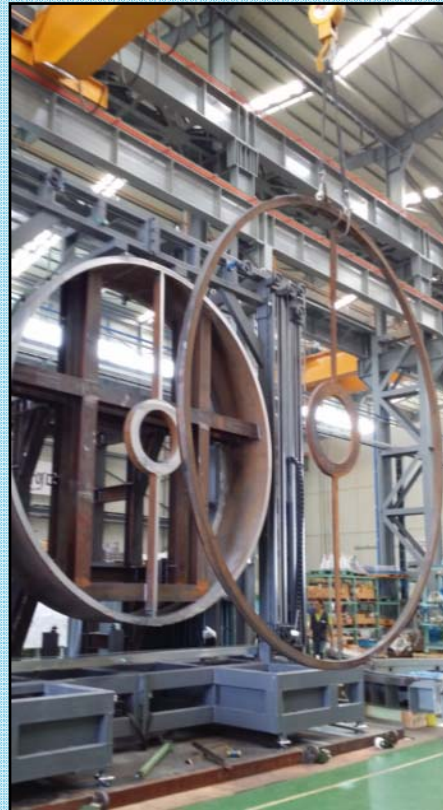
[ View after cutting ]
