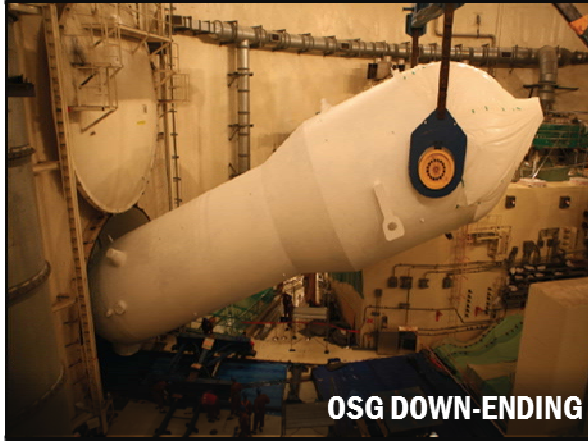
Fixture Installation & OSG DOWN-ENDING
