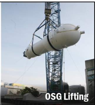
Fixture Installation & OSG DOWN-ENDING
