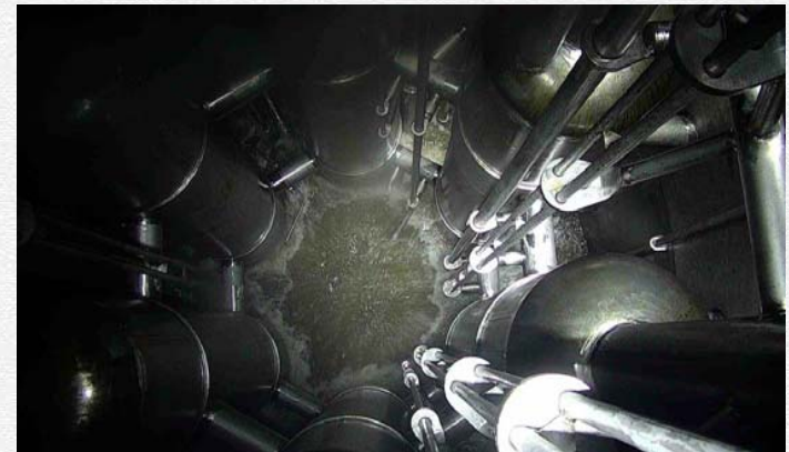
Testing of Standard High-Solids Vessel (SHSV) Initiated on Dec. 22, 2016
