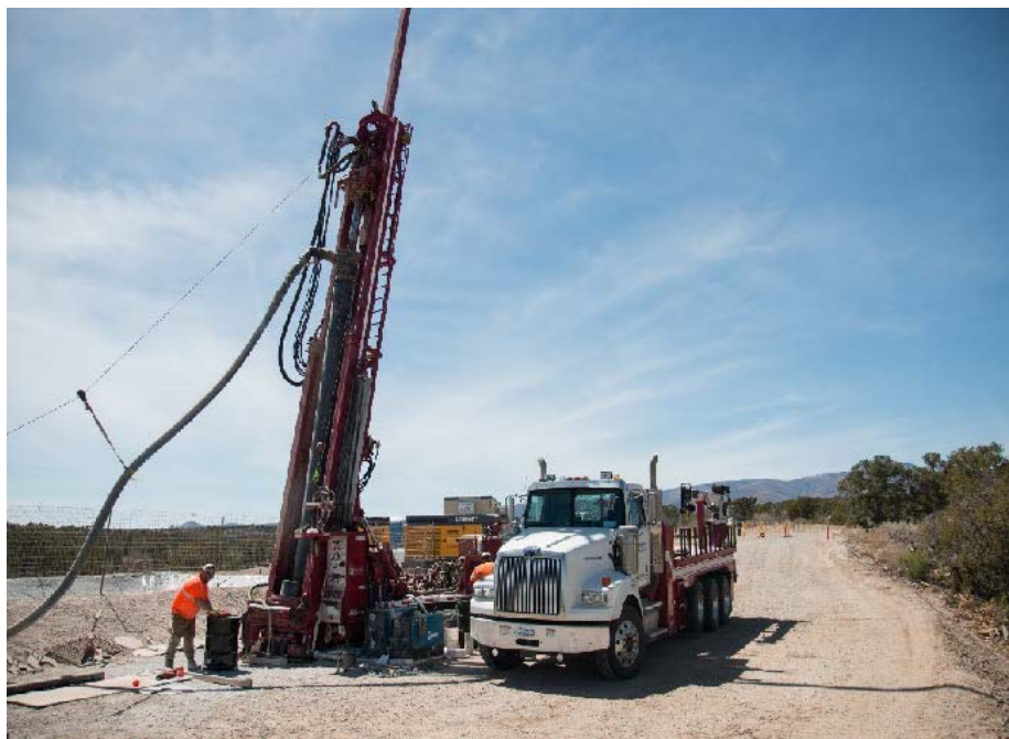
An angled drill was used to install the injection well CrIN-4 for the Chromium Project
