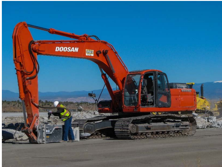
Debris being cleared at the Los Alamos County Airport landfill
