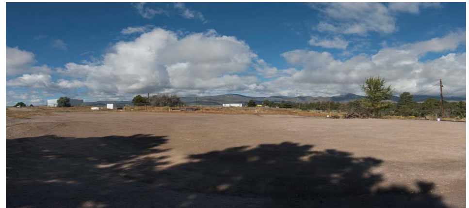
The footprint of TA-21-286 after demolition
