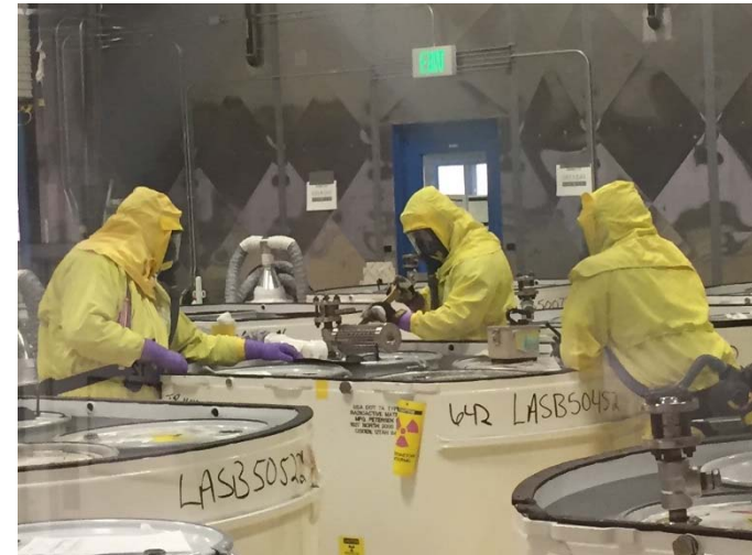
Workers installed PRDs on the RNS drums in the spring of 2016.
