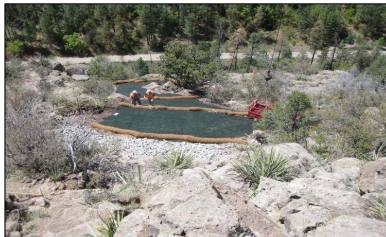
Restoration work at TA-32
