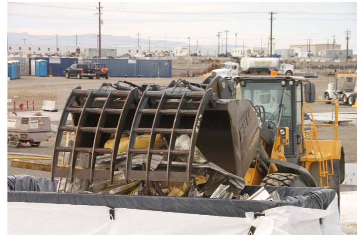
Demolition waste load out.
