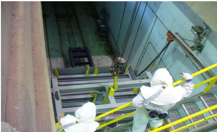
Platform being lifted in tunnel for cell placement in T Plant.
