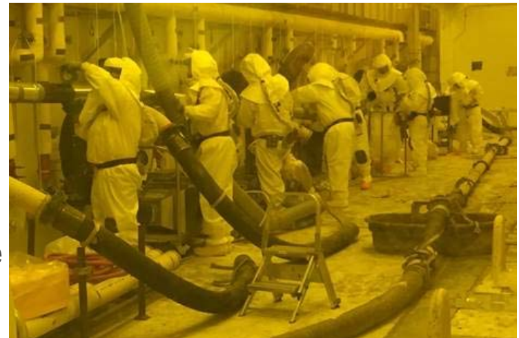
Crew in WESF canyon reinforcing temporary ventilation header.
