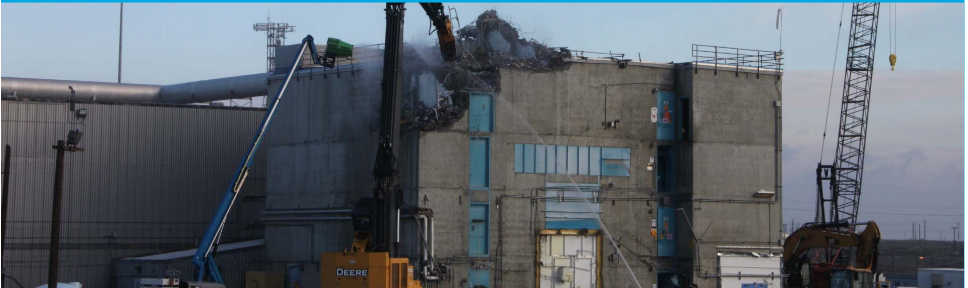
Demolition at the Plutonium Finishing Plant.
