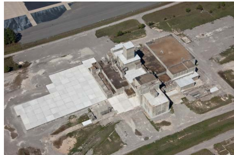
In situ decommissioning of SRS R-Reactor
