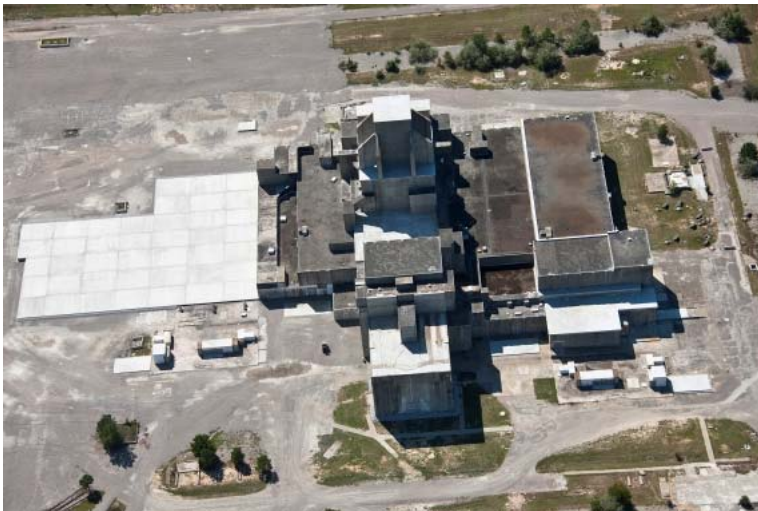
In situ decommissioning of SRS P-Reactor
