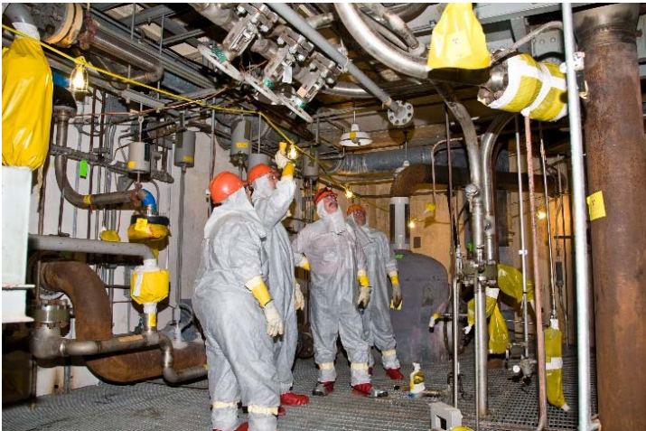
Decommissioning SRS Heavy Water Components Test Reactor
