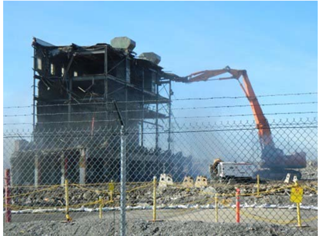
Oak Ridge ETTP, Bldg K-25 Demolition, 2014
