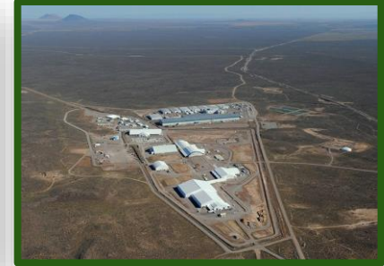
AMWTP at Idaho
